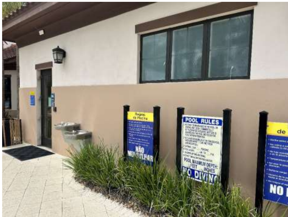
Exterior Pool Area Walls
